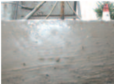
Coating of wet slurry on the edge First application of sealant
