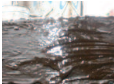
Coating of wet slurry on the edge First application of sealant
